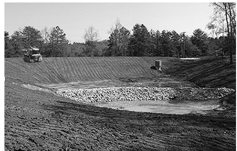
Retention Pond Under Construction
