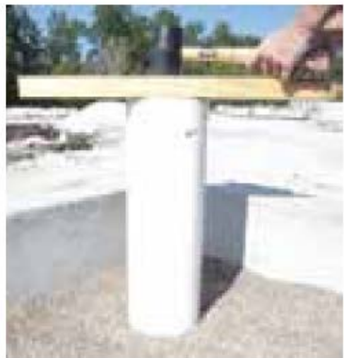
Figure 3: Hammering Pipe Into Media
