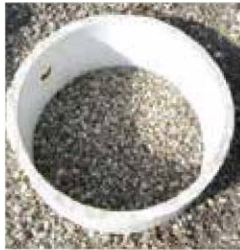
Figure 4: Pipe Installed Into Media
