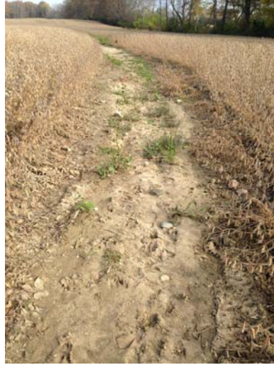
Unvegetated drainage swale
